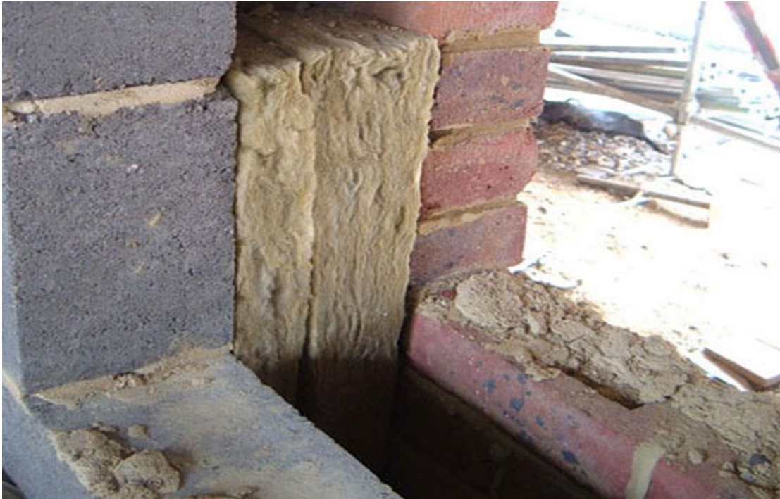
Figure 3 – Fiberglass as wall insulation reduces and minimizes heat loss in winter and prevents heat gain in summertime through walls and simultaneously, prevents sound transmission inside and outside the building.
