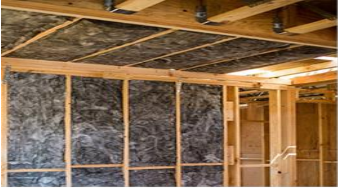
Figure 2- Fiberglass insulation in wall
