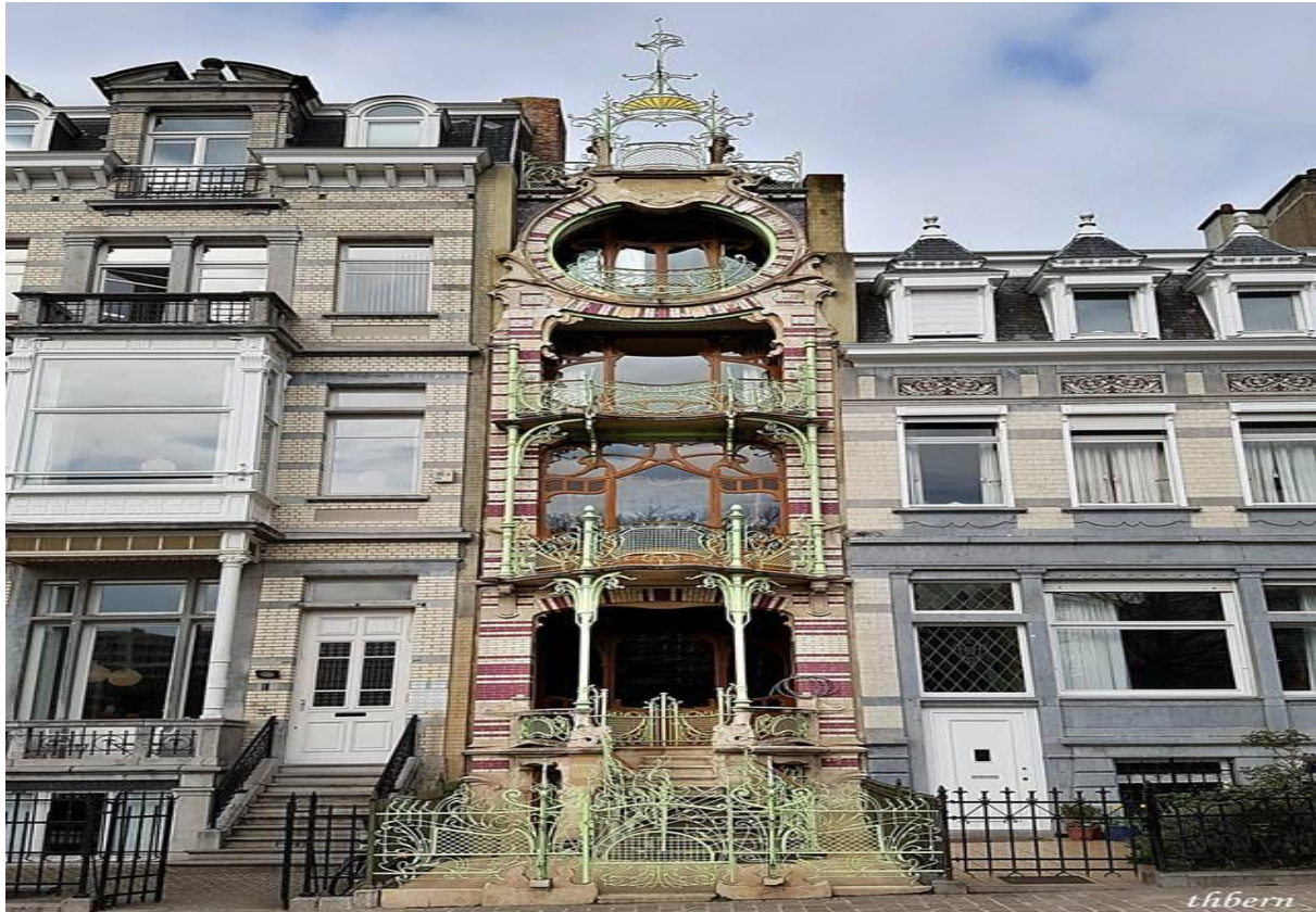
Figure 17 - The Maison Saint Cyr square Ambiorix 11, Brussels, Belgium, Architect Gustave Strauven – 1901-1903
