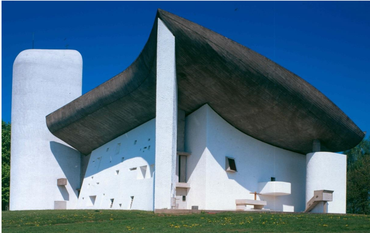
Figure 23 - Notre- dame du Haut, Roman Catholic chapel in Ronchamp, France – Architect Le Corbusier - 1955
