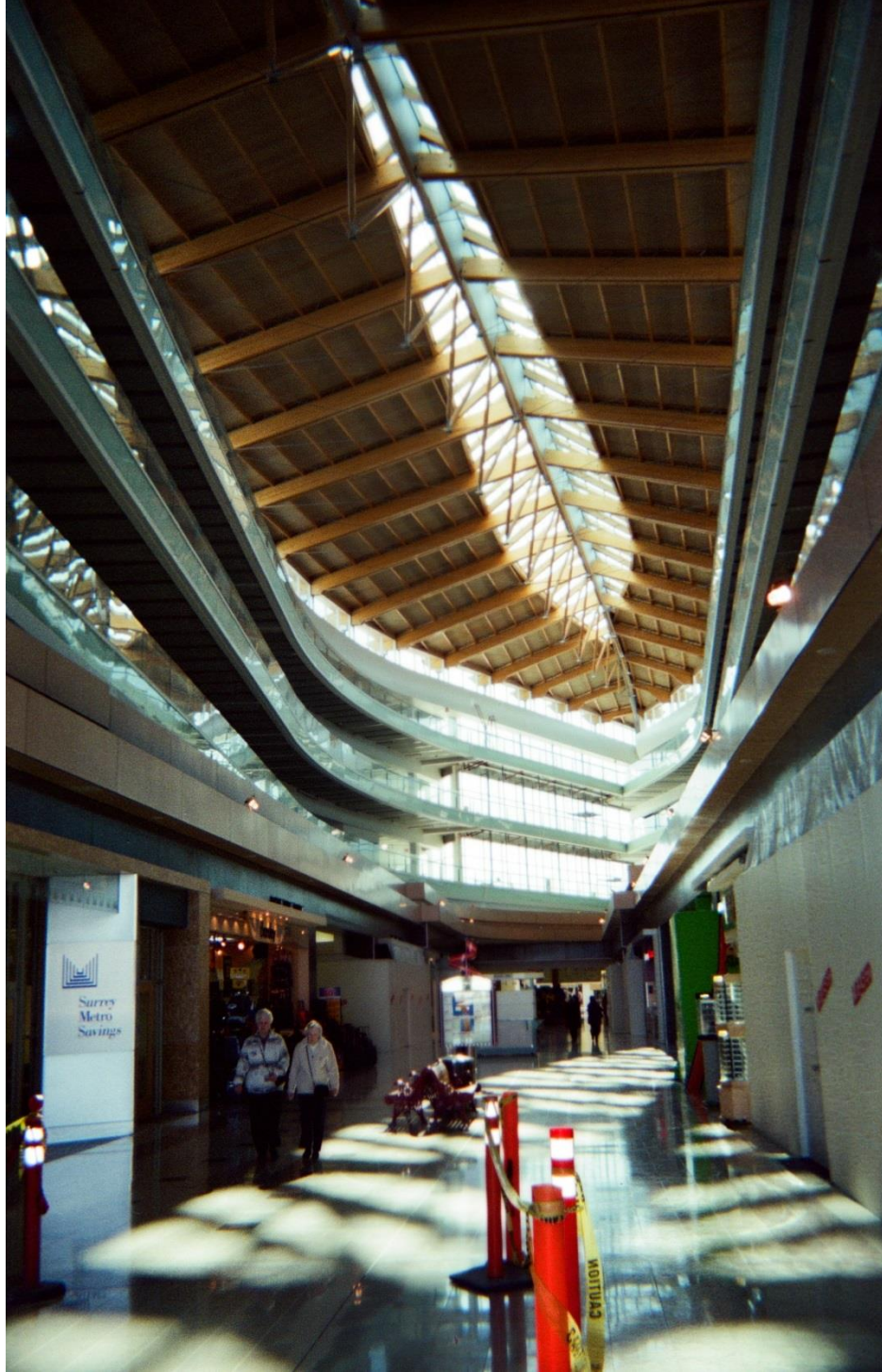
VI - The galleria's ceiling is made of a staggering wooden structures, the ceiling is astonishing and mimics shark ribs. (Photo, by Author Hossainy)
