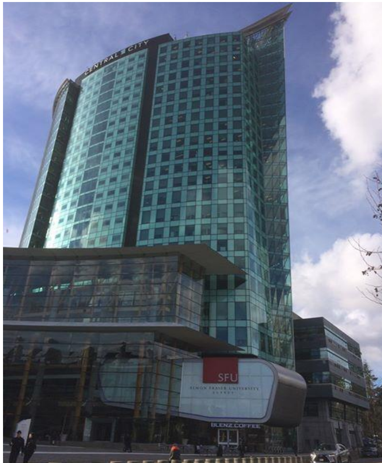
I - Northern Tower view (Photo, by Author Hossainy)
